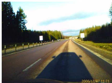
FIGURE 2 | Drying effect on a highway road. The right lane is dry because of the heat and air mixing from running vehicles. The left lane is wet because less trafficked [5].
